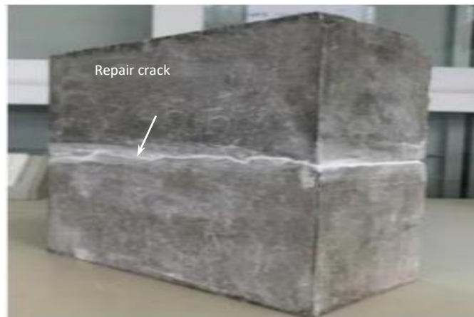
Figure 5. MICP cemented joint specimen
