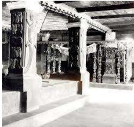
Plate 9: Carved beam and lintel at old Alaafin of Oyo and Olowo of Owo palaces.
